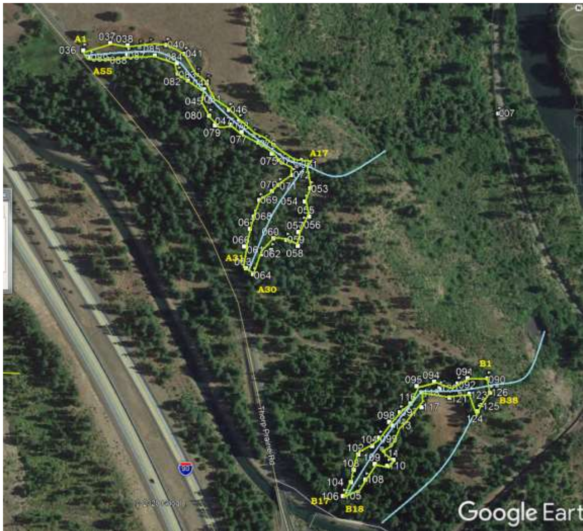
Above: Preliminary GPS mapping of Wetland A on the north, and Wetland B on the south of Area #2.
